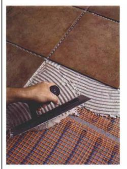
Electric floor warmers, such as this one manufactured by Bask, install easily. They use about as much energy as several light bulbs and raise the floor about  $\frac{1}{2}$  in.
